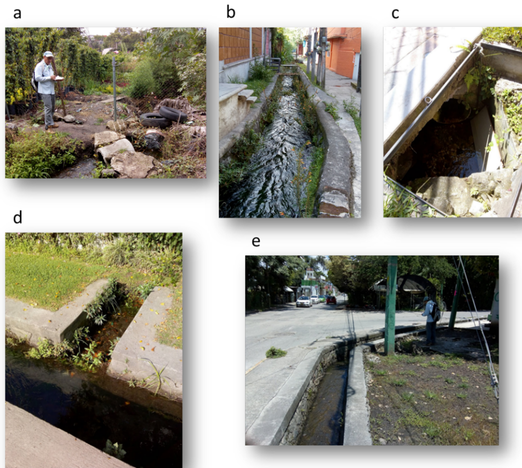
Figure 3. Images of different types of channels registered in the apantli network, Jiutepec, Morelos, Mexico. a) Earth channels in nursery areas; b) cement channels; c) PVC and/or concrete pipes; d) Canceled channels; and e) cement and stone channels. (Jaramillo Monroy et al. 2019).
